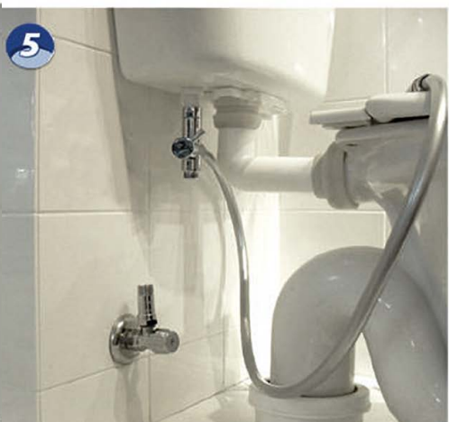
5 Fit water diverter to Cistern, ensuring you Insert Black Washer.
